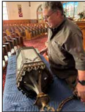
Trustee Eric Brunner repairs two ceramic bulb sockets in a chandelier
