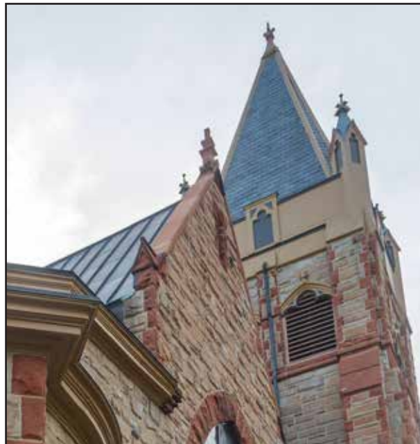
Main Street gable showing new coping stones and finial; tower stones replaced or chiseled
