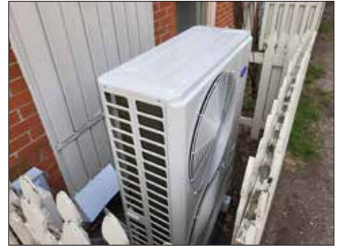
New Carrier air conditioner and heat pump
