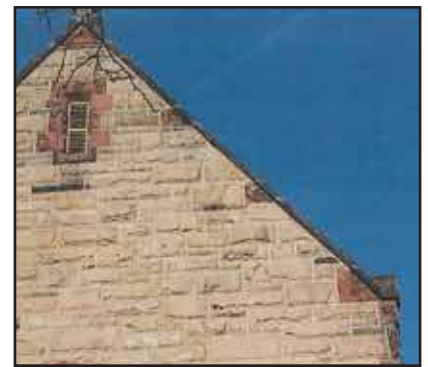
Photographs above and below showing eroded coping stones on the Main Street gable
