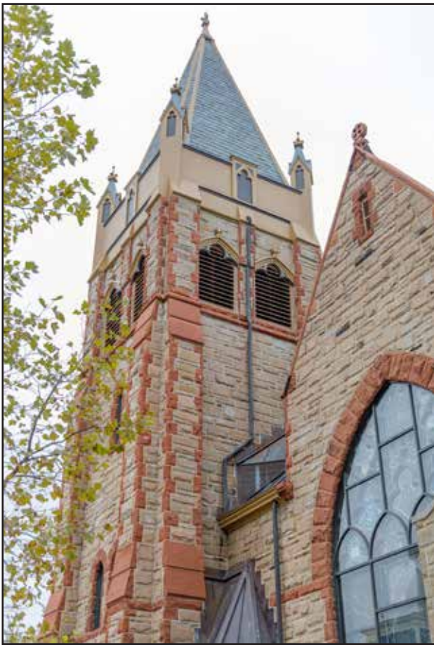
Fourth Street tower with newly installed louvers and storm window on its sanctuary window
