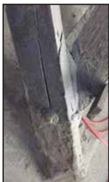
Rotten, split beams on the chime rack; it would have eventually failed because the tower roof was leaking
