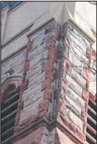
Photographs above and below showing deteriorated stones and failing mortar joints
