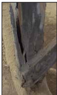
Rotten, split beams on the chime rack; it would have eventually failed because the tower roof was leaking
