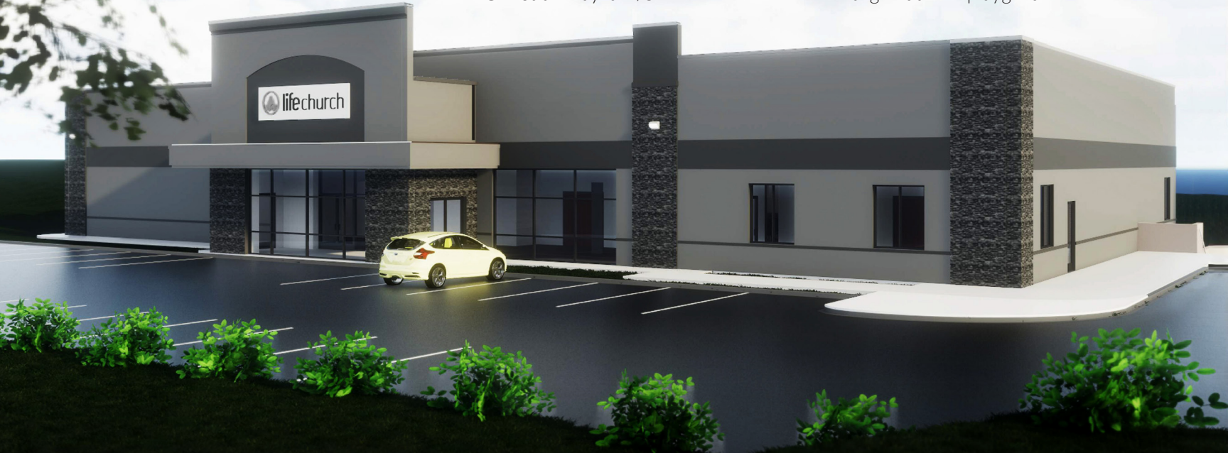
Frontview render of the Life Church Calvert building after Phase 2.
