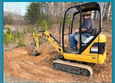
Brian clearing trees and grading land
