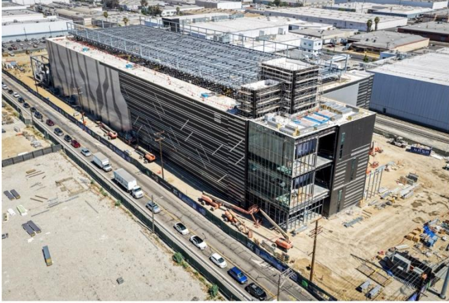
An aerial view of a 49.5 megawatt three-level data center under construction on July 8, 2026 in Vernon, California. (Mario Tama/Getty Images)
