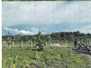
Putting up the poles in Bwera
