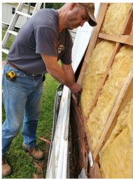
(replacing rotted structural wood on a mobile home)
