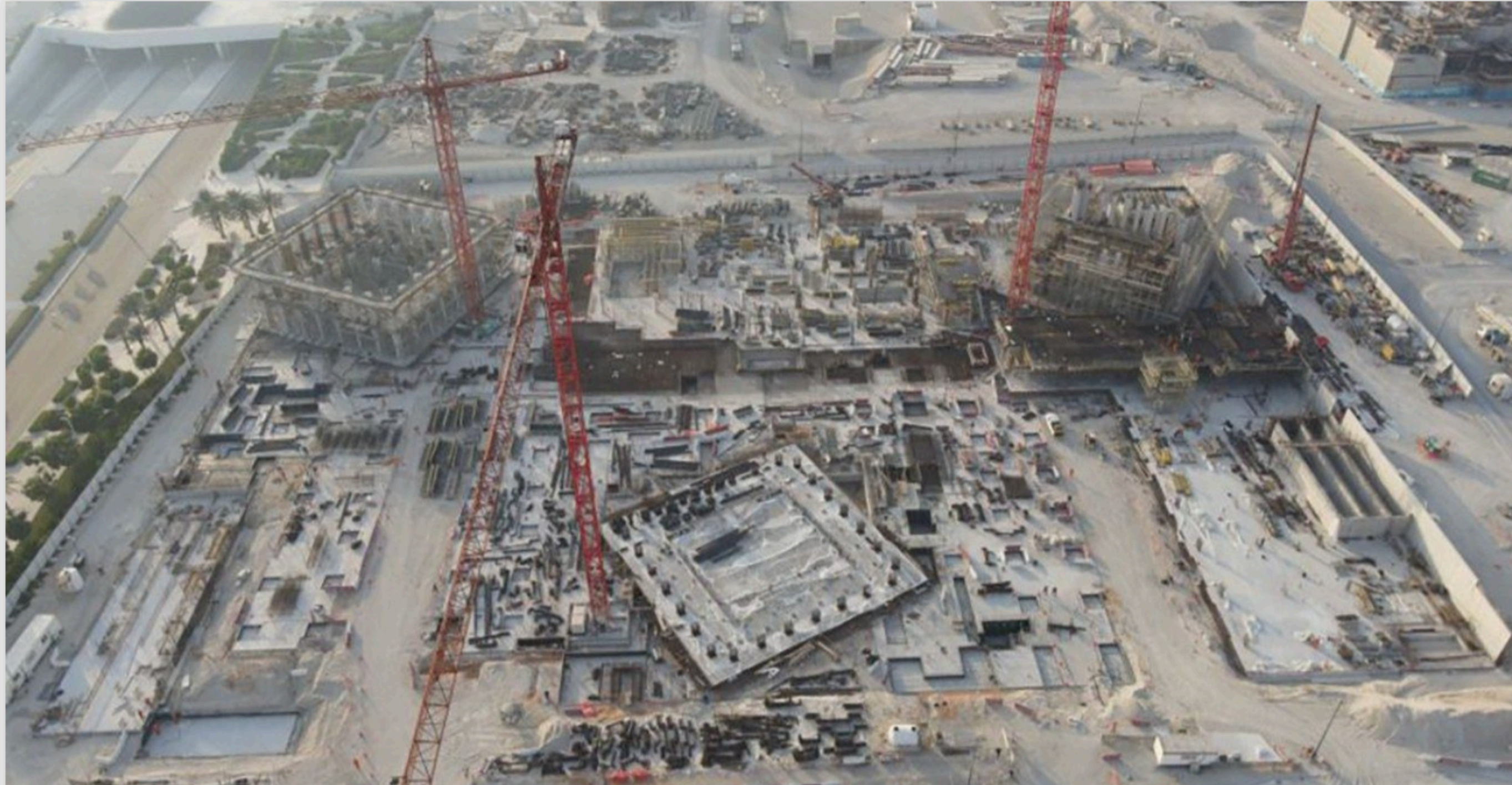
Abrahamic Family House under construction
