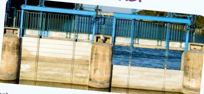
Most modern cities have floodgates that prevent destructive waters from washing away homes and other buildings. Floodgates are also used to protect farmland from being flooded and ruining crops. A floodgate is an adjustable wall or gate that can be used to control water flow for streams, rivers, flood barriers, or levees. When someone says, "open the floodgates," they are saying that they are ready for an outburst or a large flow to come forth.
